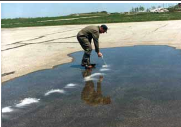
Chemical repellents, such as methyl anthranilate, can be applied to temporary pools of standing water on airports to repel birds until the water evaporates. The preferred long-term solution is to improve drainage to avoid standing water after significant rain events (photo courtesy USDA).
