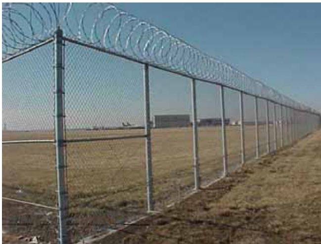
A well-maintained fence, at least 10-feet high with no gaps at the bottom, is the primary defense to keep deer and other large animals off of the AOA at airports. Gates must also be close-fitting, and water drains under the fence must be equipped with exclusion devices (top photo by E. Cleary, FAA).
