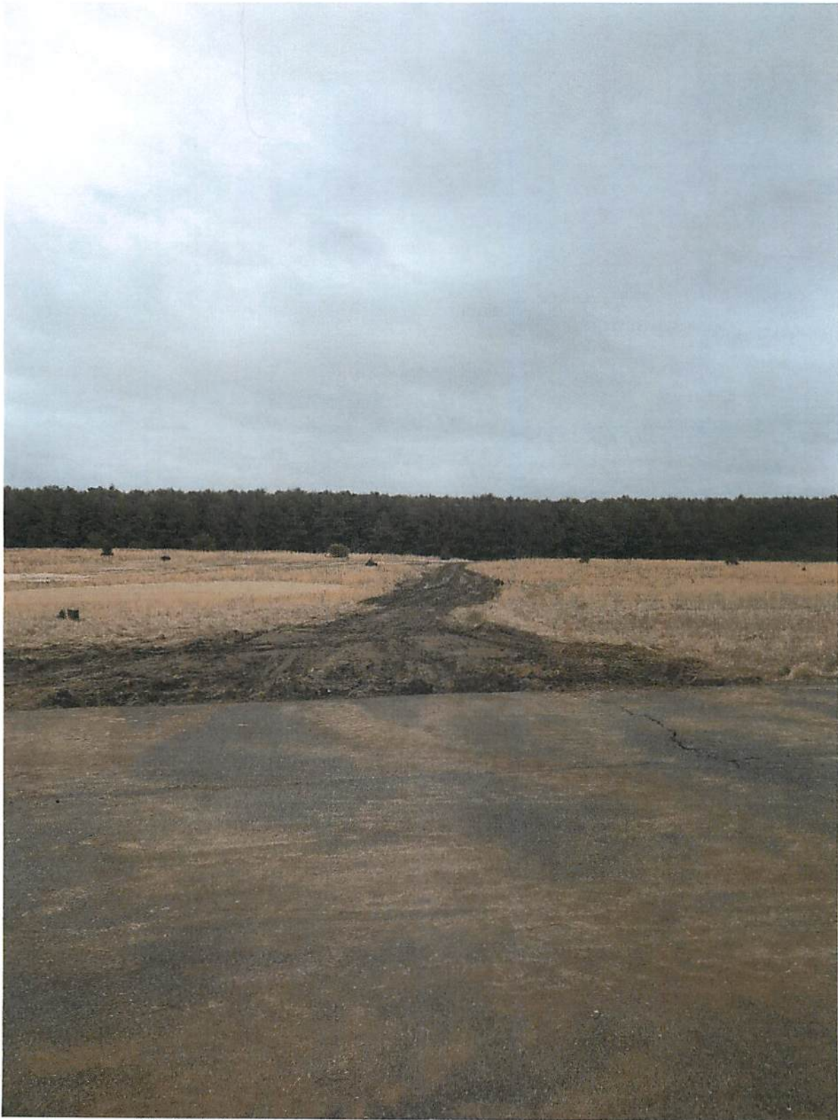
10,000 FT (East) Runway: looking East- Sewer Construction Feb. 19, 2020 40°54'45"N 72°46'36"W
